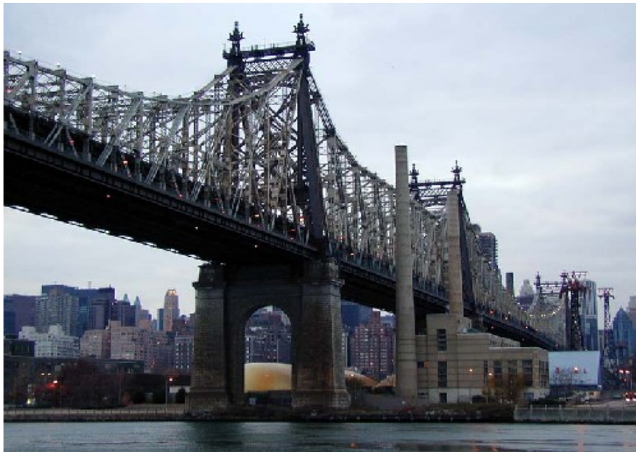
Ed Koch Queensboro Bridge (59th Street Bridge) (Gustav Lindenthal, Leffert L. Buck, Henry Hornbostel, 1909)
